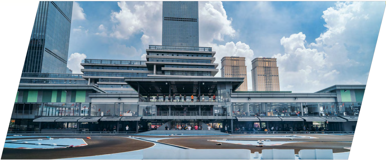
Newly built state-of-art 3 storey complex consisting of 3 tracks
